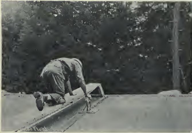
Fig. 4.—Divided float in use at expansion joint.
